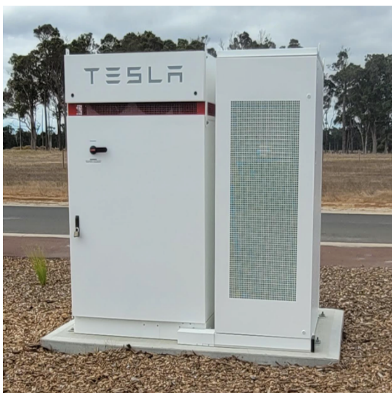
Figure 5. Cluster 1C's TESLA Powerpack
