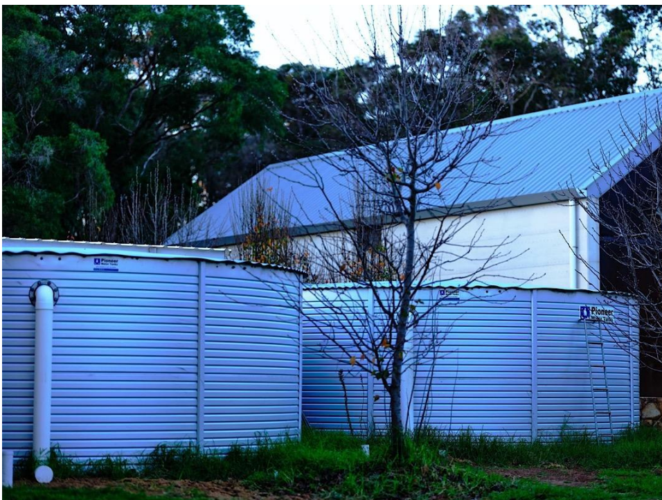
Figure 11. Rainwater tanks, Margaret River Econcepts house.
