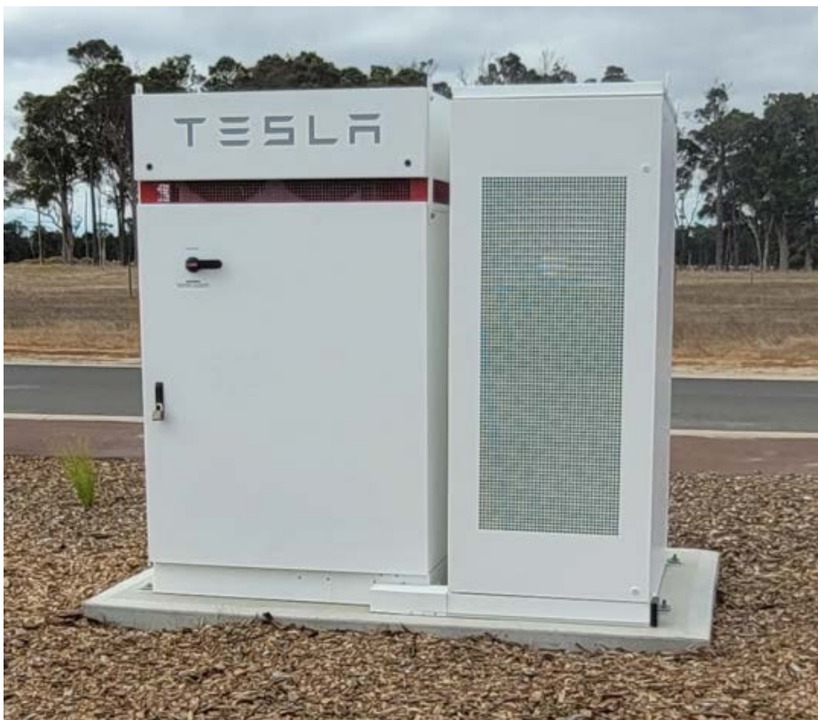
re 5. Cluster 1C's 232kW TESLA Powerpack.
