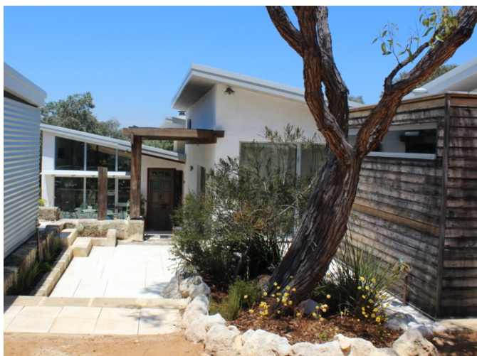
R+H Strawbale House, Sorensen Architects
